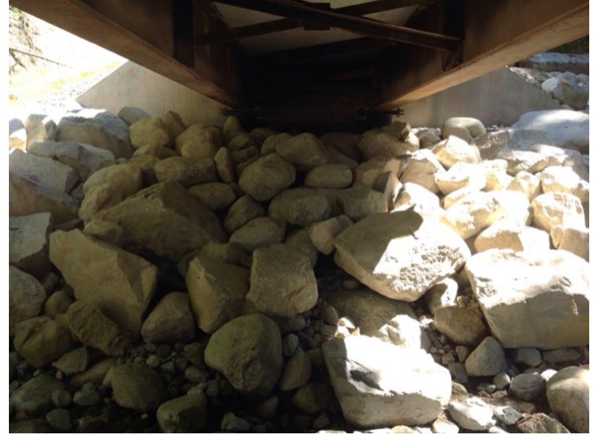
Left Bank Abutment when facing downstream
