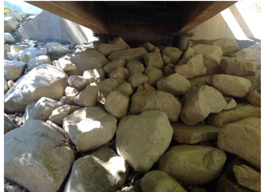
Right Bank Abutment when facing downstream
